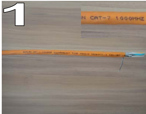
1 Strip approximately 40mm the cable jacket, fold back the foil and the braid shield
